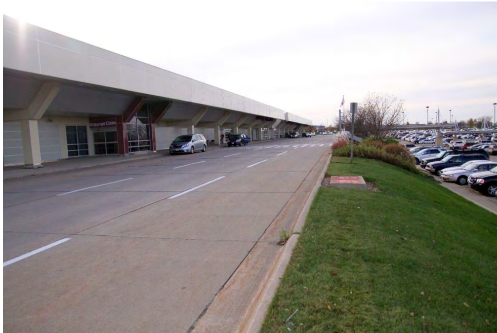
Main terminal façade and entry at the passenger terminal drop-off and pick-up area Photograph by Mead & Hunt, Inc. (2011)
