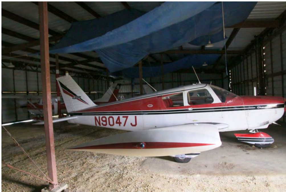
Interior of one of the West T-hangars. Note the gravel floors and tarp covering a leaky roof. Photograph by Mead & Hunt, Inc. (2011)
