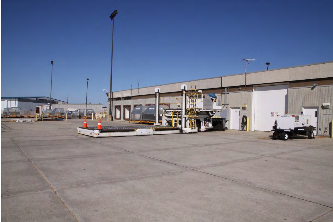
Exterior of UPS/USPS Cargo Distribution Facility Photograph by Mead & Hunt, Inc. (2012)
