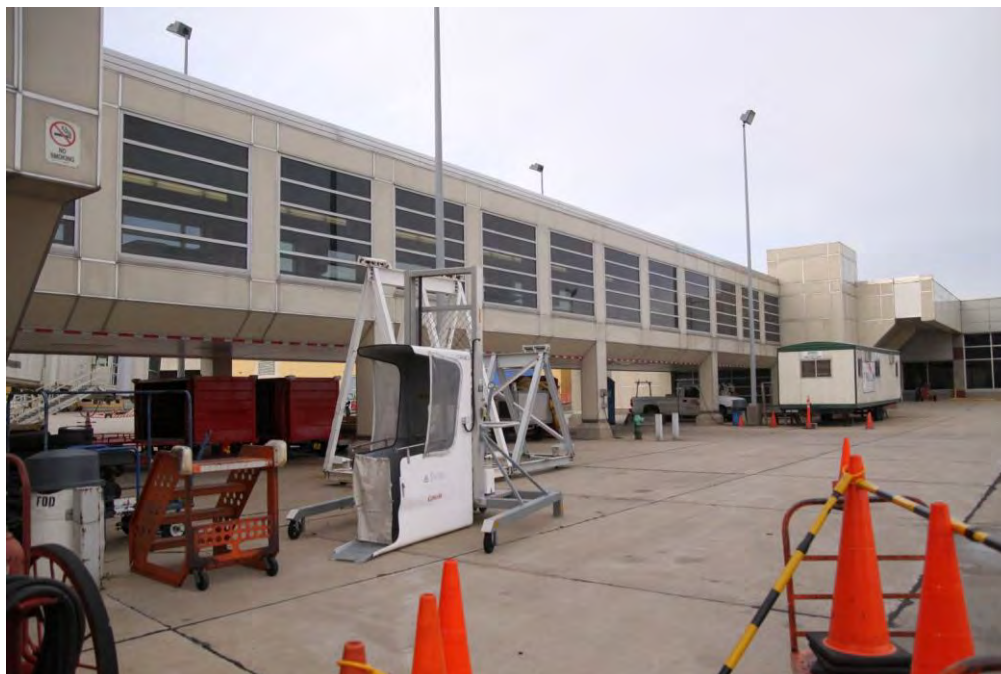
Area under the Concourse 'C' walkway that is currently used for GSE storage Photograph by Mead & Hunt, Inc. (2011)
