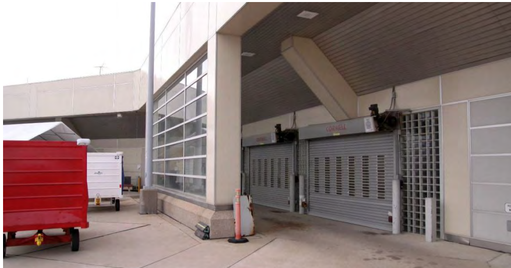
The Eastern Iowa Airport passenger terminal inbound baggage area Photograph by Mead & Hunt, Inc. (2011)
