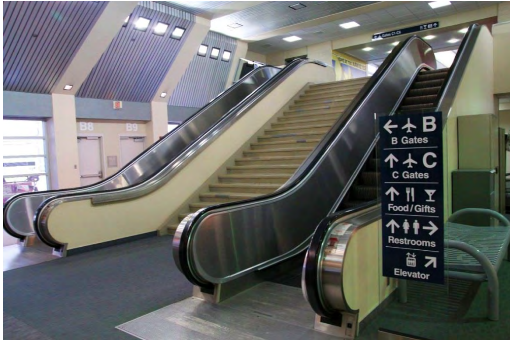
Escalators and stairs provide access to upper level and Concourse C Photographs by Mead & Hunt, Inc. (2011)
