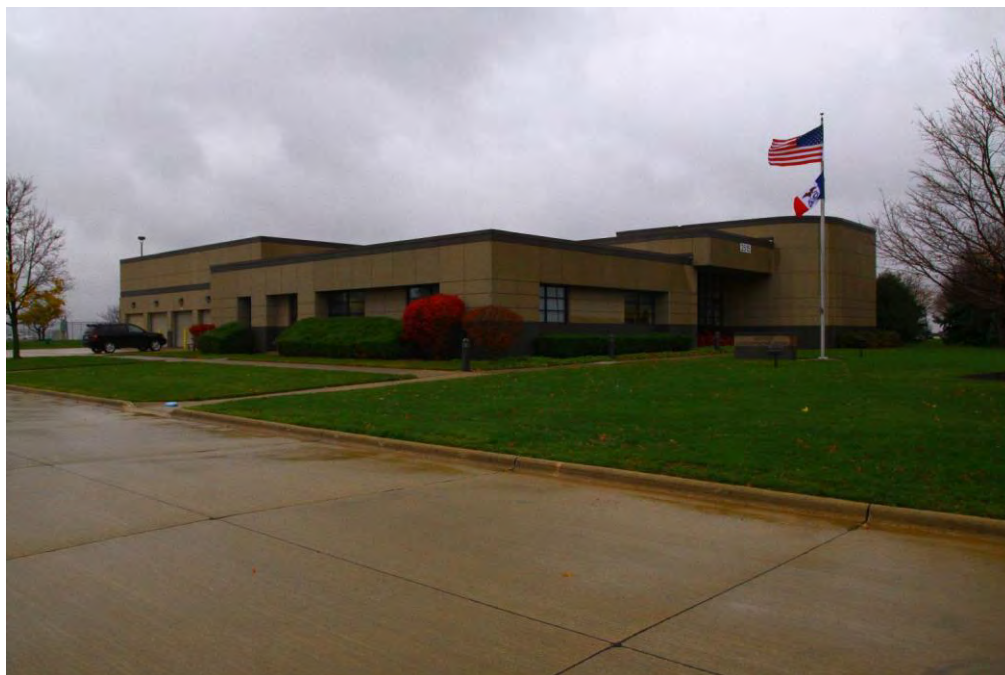
Administration building Photograph by Mead & Hunt, Inc. (2011)
