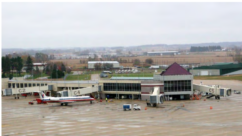
CID terminal building C Concourse Photographs by Mead & Hunt, Inc. (2011)
