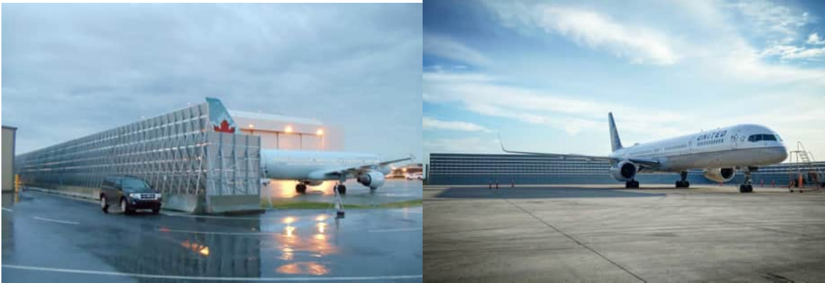
Figure 4.13: Ground Run-Up Enclosures
