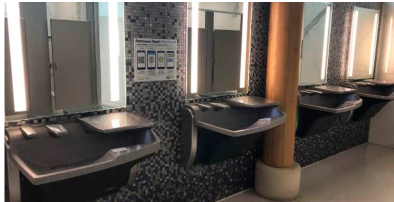
Low-flow sinks and sensor-operated faucets in terminal restrooms
